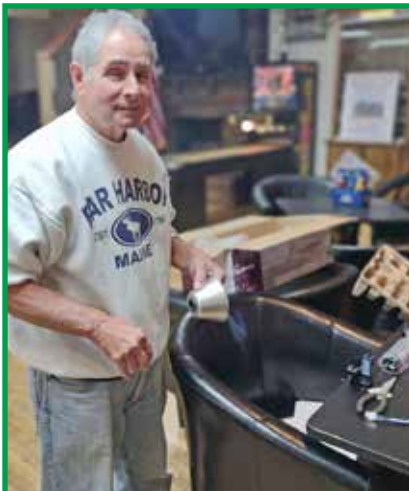
Paul Hawkins unpacking a fan to be installed in the ceiling.
