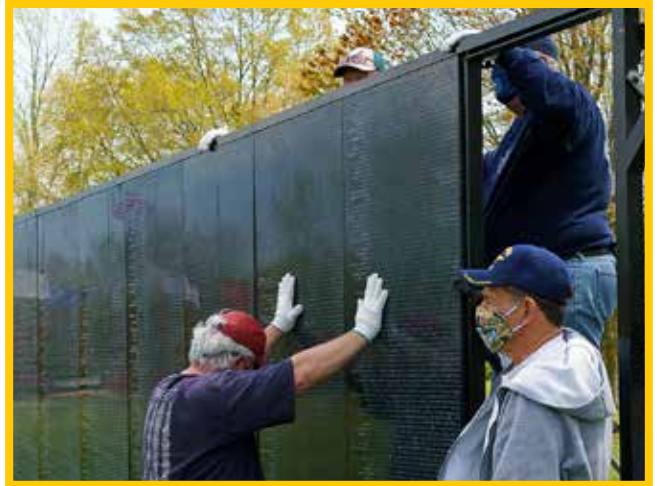
Another panel put in place
