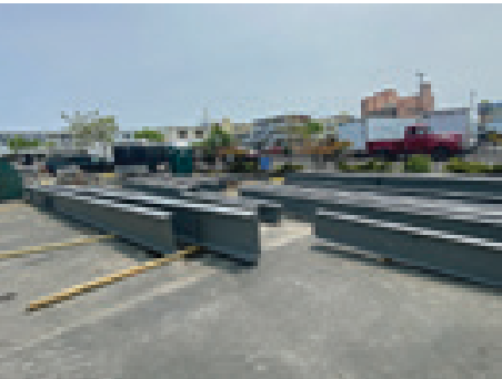
Delivery of steel beams for to support the floor
