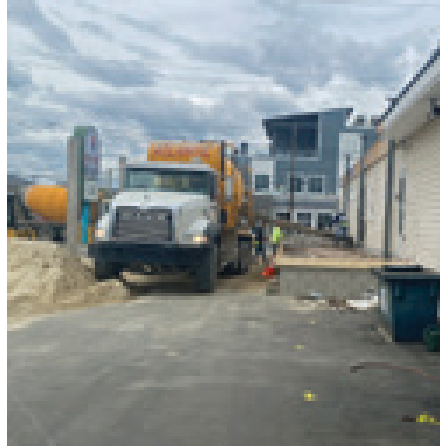
In come the trucks to take out debris
